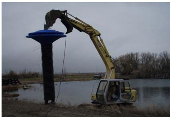
**Figure 3.** Radial flow Bluefrog™ pump
