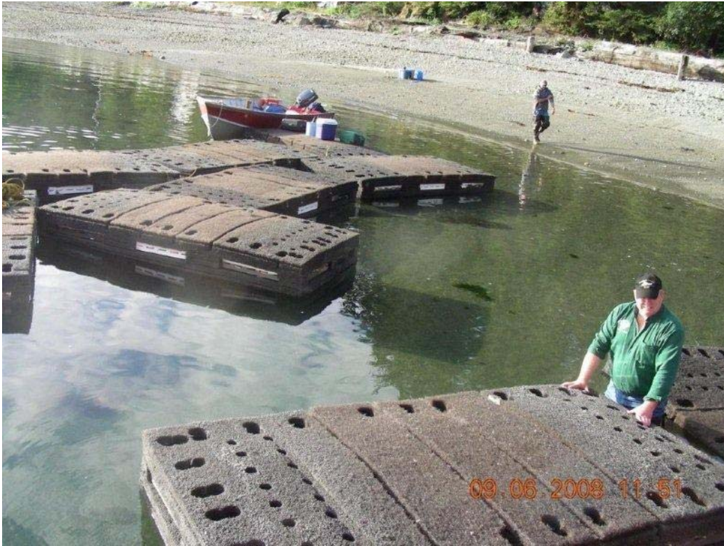
Installing the BioHaven® modules
