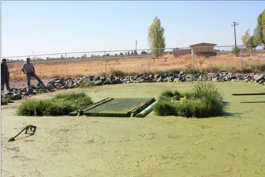
The BioHaven Streambed FTW shortly after installation in August 2012
